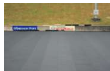
The NHS Turf replacement is well underway. Old turf all gone now; the shock pad glued in place and the new carpet is here ready for installation in January.
