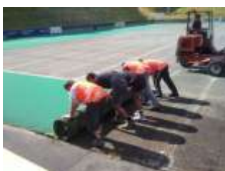
The NHS Turf replacement is well underway. Old turf all gone now; the shock pad glued in place and the new carpet is here ready for installation in January.
